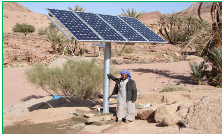
Water Pumping (Egypt)
